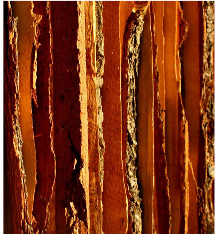
Figure 4: Reclaimed bark rainscreen siding. (Detail) (Image: Author)
